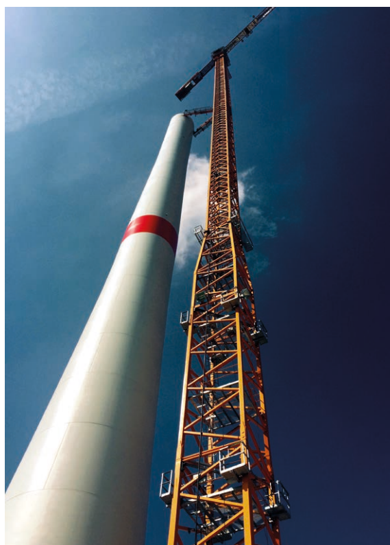
Figure 1 Hybrid tower made of prefabricated concrete elements
