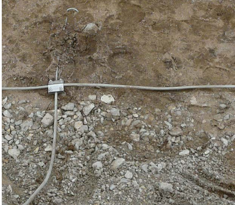
Ringerder, Rundstahl, NIRO V4A
