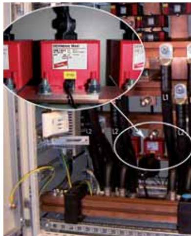
Fig. 8.1.6.5 DEHNbloc Maxi S: coordinated lightning current arrester for the busbar with integrated backup fuse
