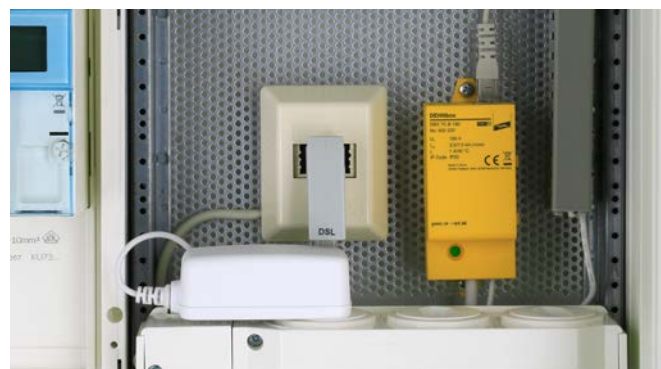
DEHNbox used for a telecommunication connection (example: U_{k0} interface)
