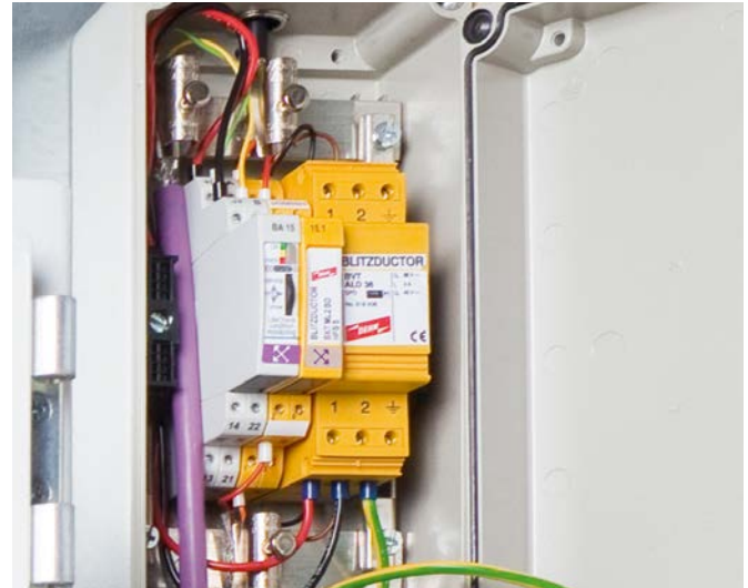
Compact DIN rail mounted surge protective device with screw terminals for stranded lines.
