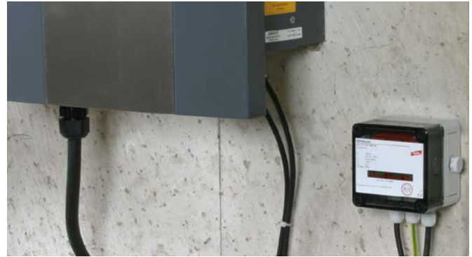
For protecting low-voltage consumer installations against surges. For use in accordance with IEC 60364-7-712 (photovoltaic (PV) power systems).
