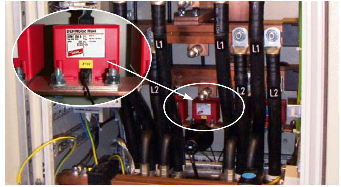
For protecting low voltage consumer installations against surges and even direct lightning strikes. For installation in conformity with the lightning protection zone concept at the boundaries from 0_A - 1 .
