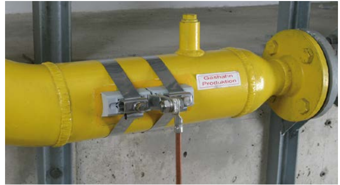
Pipe clamp for electrical contacting pipes in hazardous areas for implementing lightning equipotential bonding according to IEC / EN 62305-3
