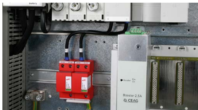
For protecting d.c. consumer installations against surges and even direct lightning strikes. For installation in conformity with the lightning protection zone concept at the boundaries from 0_A - 1 .
