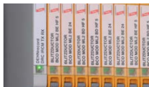
Connect = Protect Simple status message with monitoring unit for arrester groups
