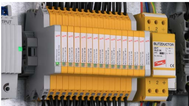
BLITZDUCTORconnect for protecting measuring and control systems
